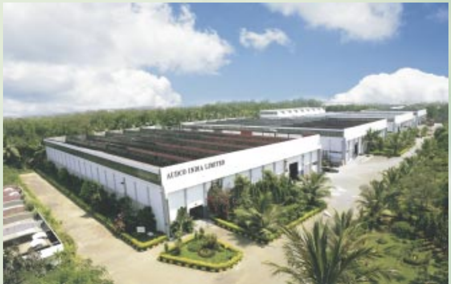
Maraimalai Nagar plant
